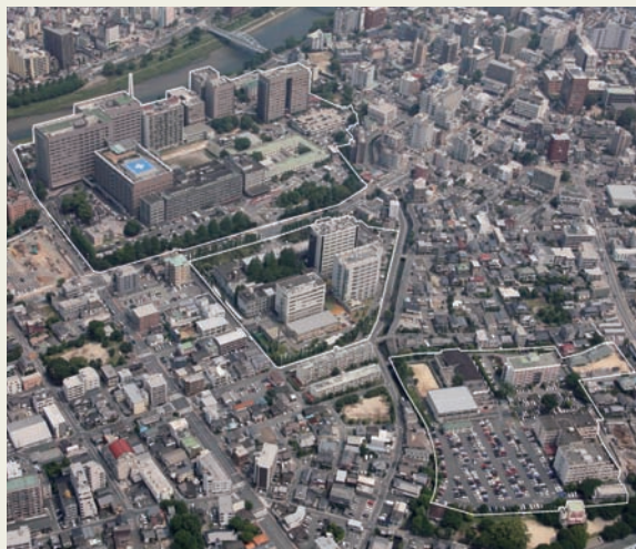
Honjo North, Center, South Campus (133, 312m 2 )
