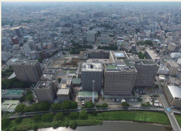
Honjo North, Central, South Campus (135,815m 2 )
